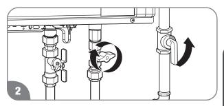
Close the gas shut-off valve(s).
