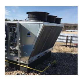
Installed DOAS unit at the Laboratory
