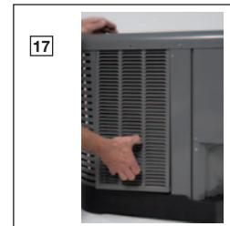
The outdoor fan motor has sleeve bearings and is inherently protected. The motor is totally enclosed for maximum protection from weather, dust and corrosion. Access to the outdoor fan is made by removing four fasteners from the fan grille. The outdoor fan can be removed from the fan grille by removing 4 fasteners in the rare case outdoor fan motor fails.
