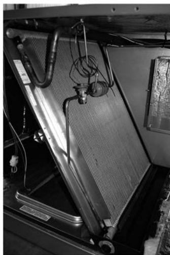
Evaporator Coil/Filter Access
