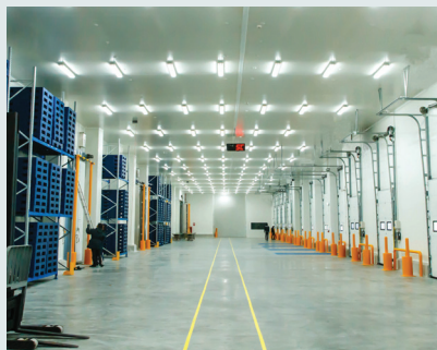
Cold Storage Warehouses
