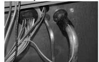
Freeze Sensor (RKKN-C Only)
