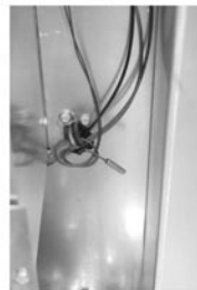
Discharge Air Sensor
