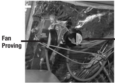
Clogged Filter Switch
