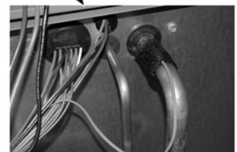
Freeze Sensor (RKKN-C Only)
