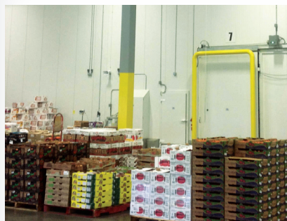
Medium to Large Warehouses
