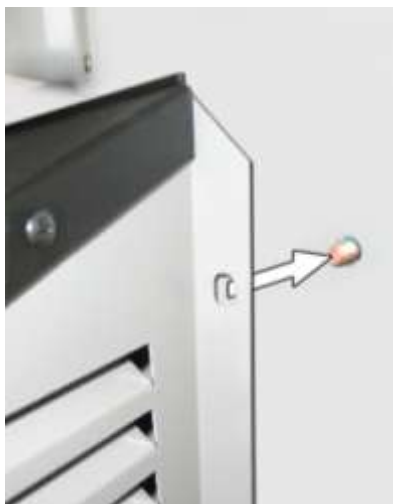
Steps 18 and 19 align heat pump module over studs and screw on flange nuts
