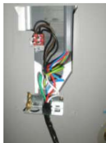
Step 3 withdraw the power cable
